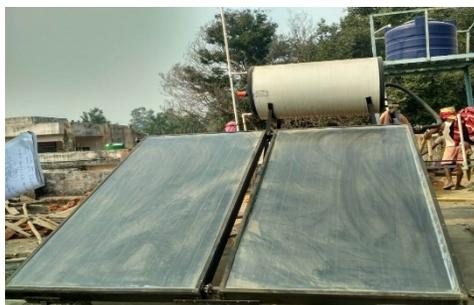
*Fig3- Flat Plate Solar Water Heater at MED, MMMUT Gorakhpur*
