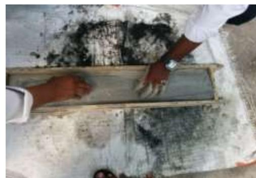
Fig.6 Placing of Reinforcement in Plate Element
